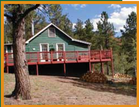
Figure 10: Decks, exterior walls and windows are important areas to examine when addressing structure ignitability. Photo: CSFS
