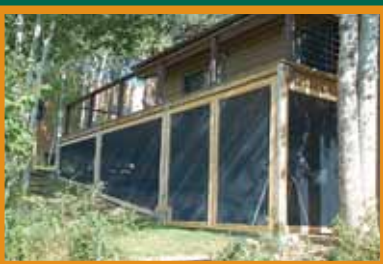
Figure 16: Enclosing decks with metal screens can prevent embers from igniting a house. Photo: Marilyn Brown, La Plata County
